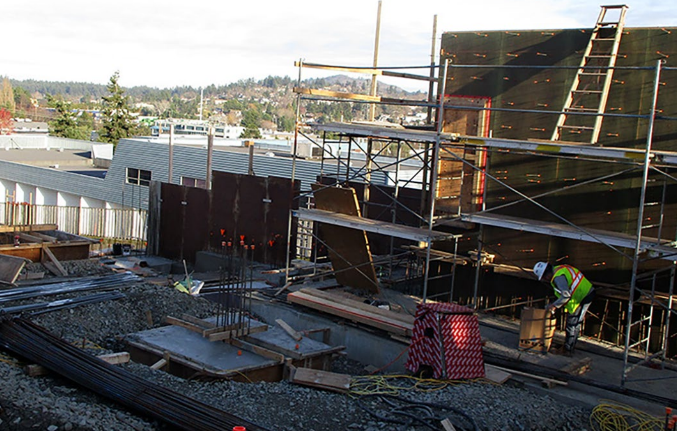
Construction of the new South Island 9-1-1/Police Dispatch Centre began in October.
